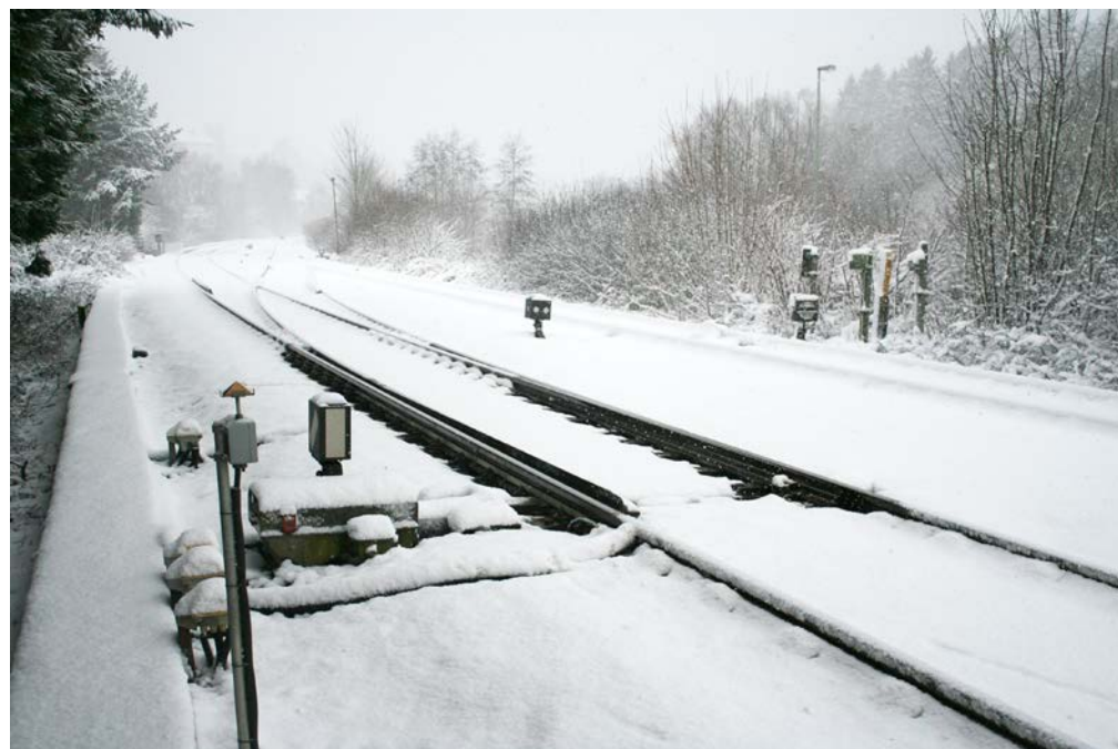
Example of a switch point heating being tested in Burbach, Germany.
